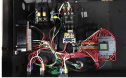
**PROGRAMMABLE SMART CONTROL** now standard for all VGH machines allows auto start/stop and time delay shutdown features without changing any hardware. It also provides complete control of the equipment run time.
